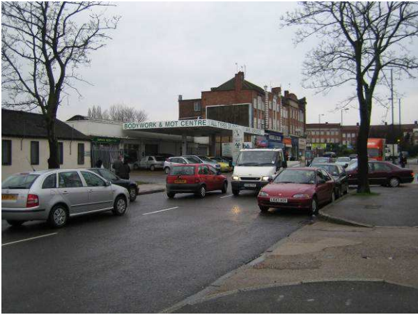
Kenton Lane – Before measures
