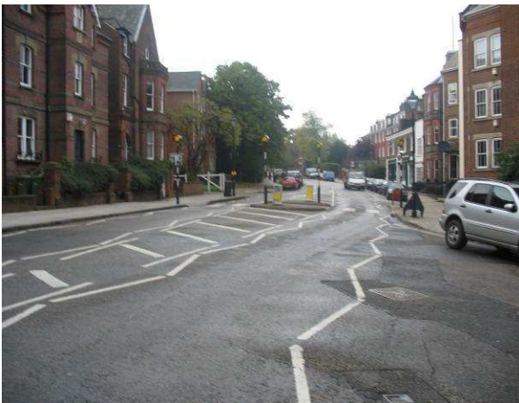
Harrow-on-the Hill – Before measures
